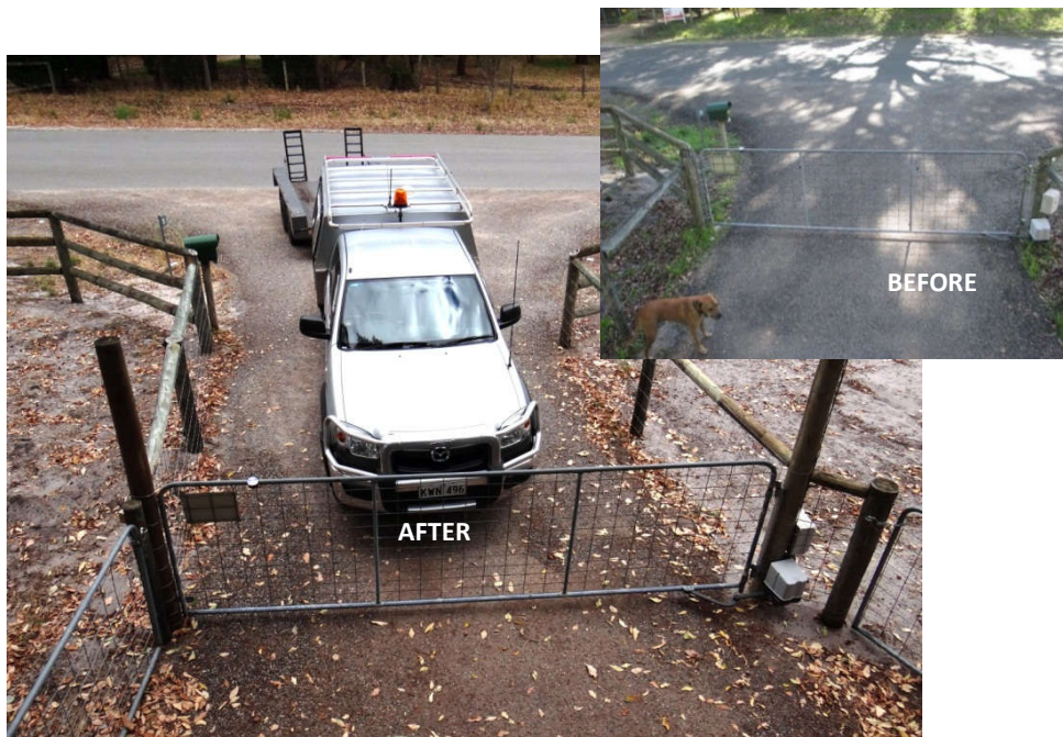
Figure 1 AFTER modifying the driveway 'lead-in', a car can comfortably pull completely off the road even with a car-trailer in tow. BEFORE modification a car could safely pull off the road but not if towing a trailer.
