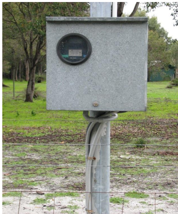
Figure 1 Locked electrical meter box, showing viewing window for meter reader to see meter information - installed adjacent to front fence for easy access.
